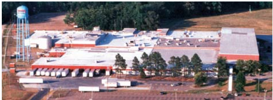
Manufacturing facility in Hamilton, NC
